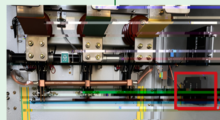
partial discharge online monitoring sensor applicable to ultra-sound, ultra-high frequency and transient ground voltage
